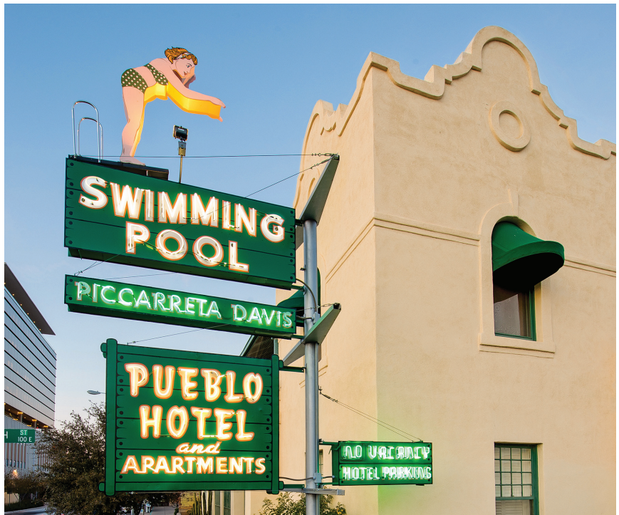
A years-long effort to restore the iconic diving girl sign on the Pueblo Hotel in Tucson prompted the city to rewrite its sign code to allow for preservation of local landmark signs.
